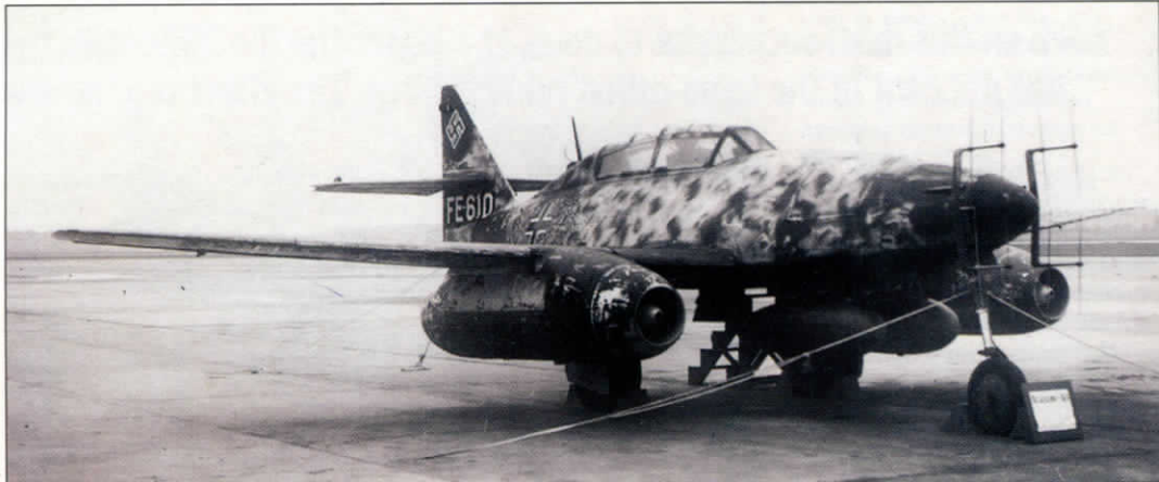
ABOVE The variant Capt Brown flew for his report on the type was an Me 262B two-seat nightfighter. This example is seen at Freeman Field in the USA after the war where it was used by Col Harold Watson and his team for USAAF evaluation.
